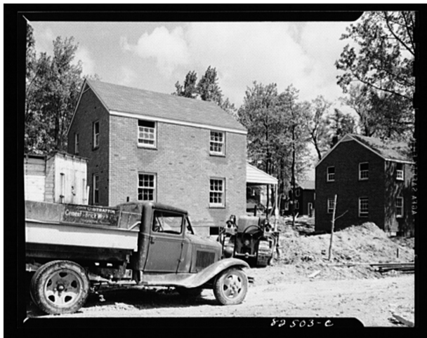
May 1942. Construction in the Greenbrier Section. Photo by Farm Security Administration photographer John Collier, Jr. Courtesy Library of Congress.
