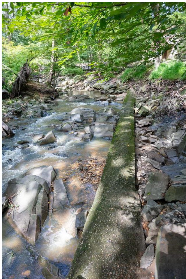
A concrete-encased sewerline exposed by erosion along Lubber Run. Photos: Dan Brown.
