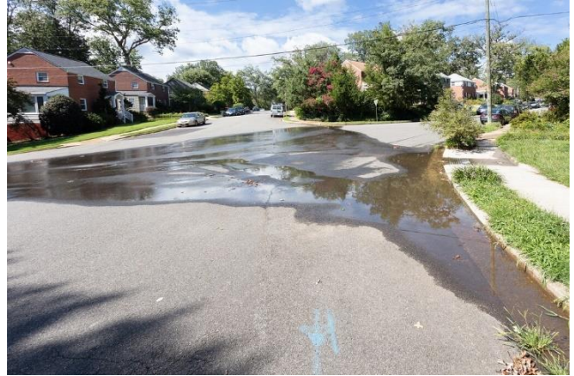
Poor drainage at the intersection of South Park Drive with South Columbus Street. Photo: Dan Brown.
