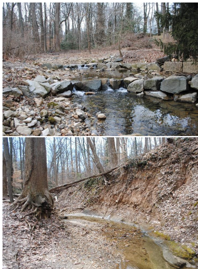
Restored (top) and unrestored (bottom) sections of Donaldson Run in North Arlington. The photos, taken well after torrential rains and flooding in 2019, suggest that stream restoration works to reconnect a stream to its floodplain and reduce erosion. Photos: Hutch Brown.
