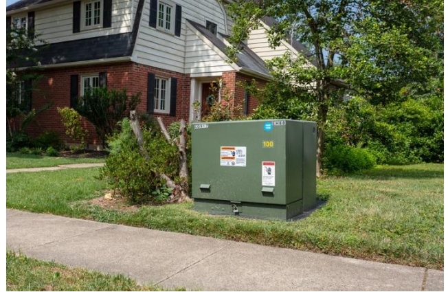
A transformer for underground powerlines in Southside, a reminder that undergrounding is possible.
