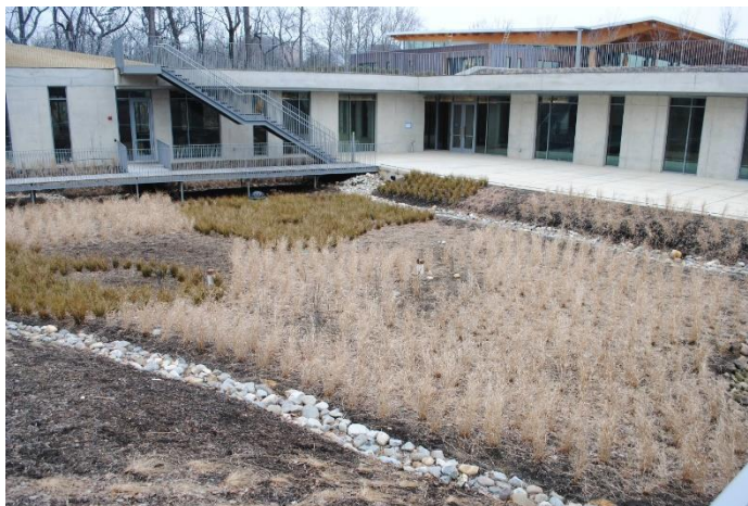
Newly installed bioretention pond at the Lubber Run Community Center in 2020. Photo: Hutch Brown.
