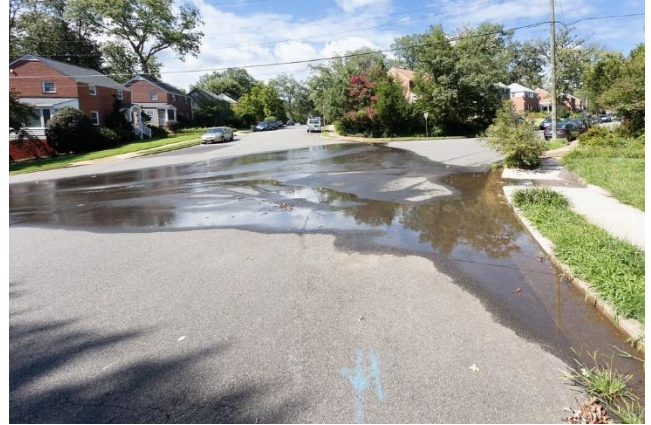
Poor drainage at the intersection of South Park Drive with South Columbus Street. Photo: Dan Brown.
