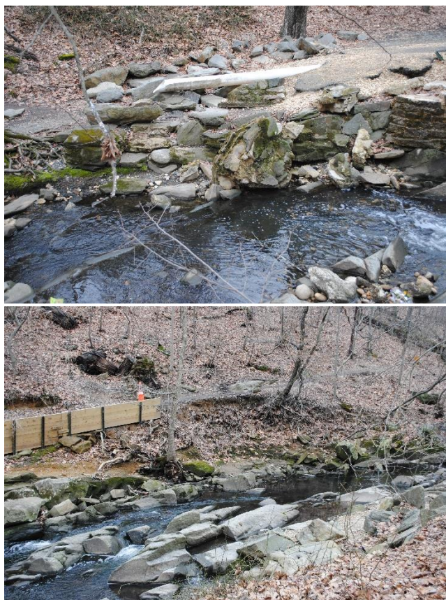
Erosion scars (top) along a popular unpaved trail in Lubber Run Park. Makeshift repairs (bottom) are vulnerable to a major storm. Photos: Hutch Brown.
